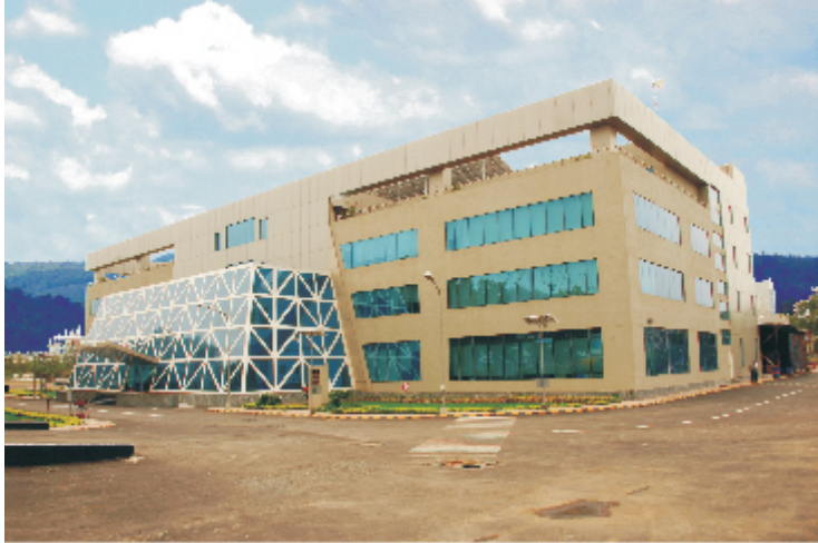
Switchgear Factory, Navi Mumbai
