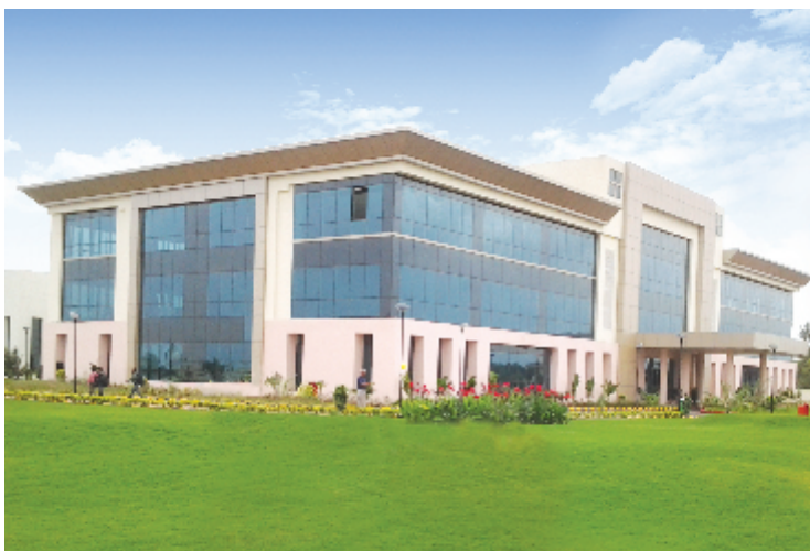
Switchgear Factory, Vadodara
