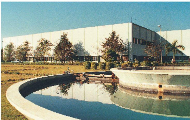
Switchgear Factory, Ahmednagar
